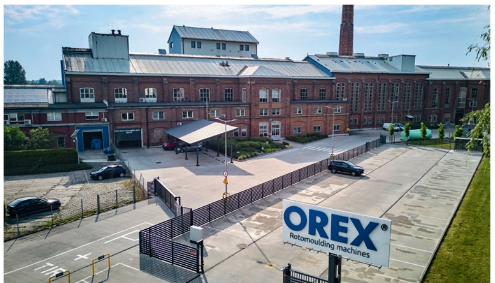
High tech concealed behind old brick walls: Over 70 highly qualified specialists work on the rotomoulding machines in the workshops extending across an area of more than 10,000 m 2 at the company headquarters in Chybie.
