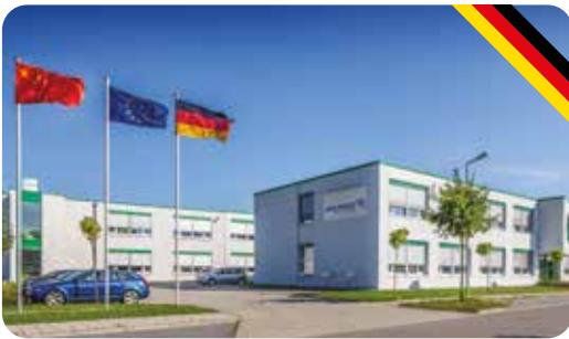
NOACK / SIEBLER, Karlsruhe, Germany
