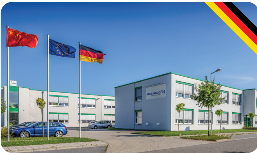
NOACK / SIEBLER, Karlsruhe, Germany
